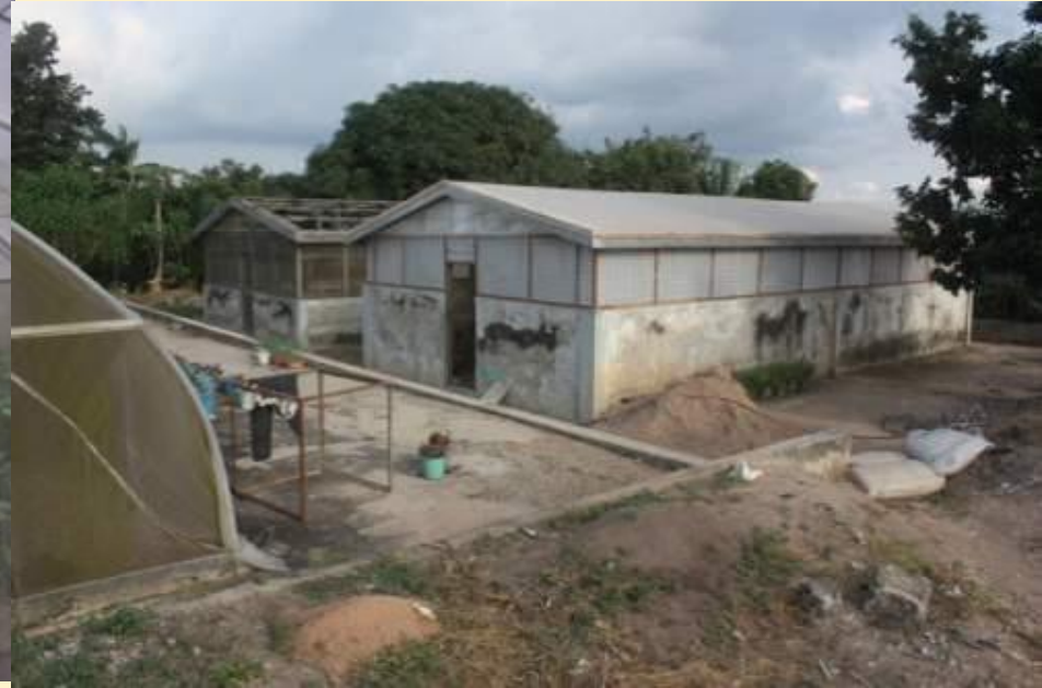
REFURBISHED HOUSE FOR GRAFTING/ QUARANTINE
