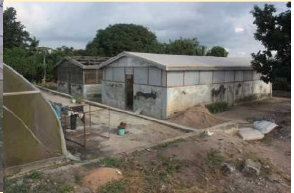
REFURBISHED HOUSE FOR GRAFTING/ QUARANTINE
