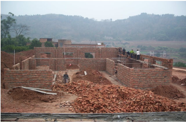
Workshop in construction
