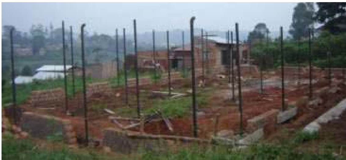
Figure 2. Foundation stage of the 200-m 2 screen house at BioCrops.
