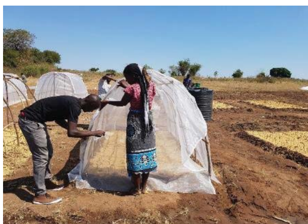
Fig 2. Net tunnel under construction in Sengerema district, Tanzania. (credit K. Ogero)
