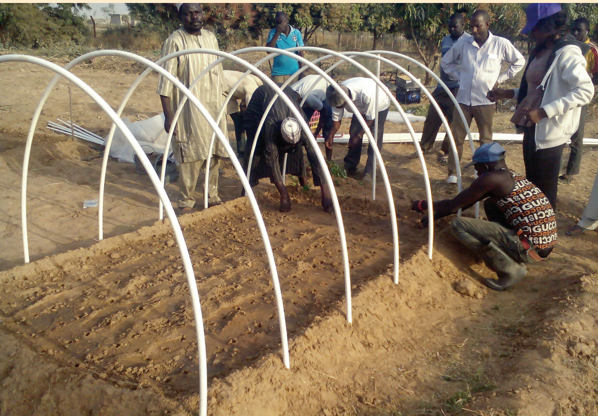
Plate 1. Constructing a net tunnel frame using PVC pipes. Nigeria. Photo credit: J. Njoku.
