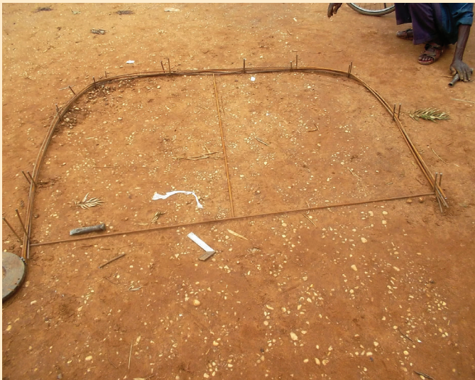
Plate 3. Bending the reinforcing rods with the aid of iron pegs planted on the ground. Uganda. Photo credit: S. Namanda.
