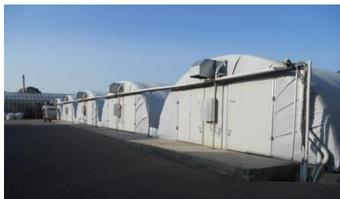
Figure 6.3 Insulated tunnel store types
