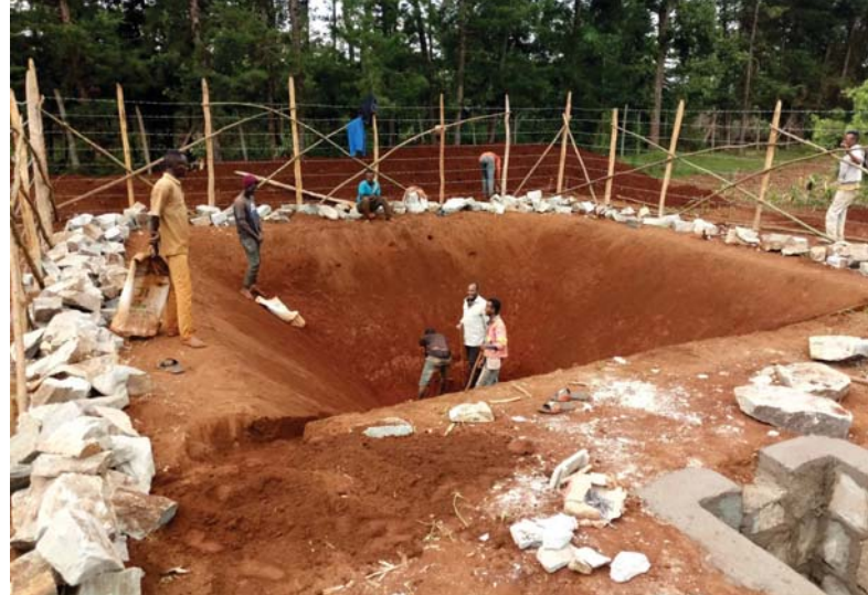
Fig 4. Construction of rainwater harvesting installation at Gure FTC (Credit: R. Brouwer)
